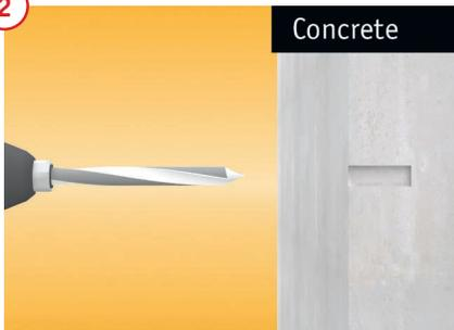
Pre-drill the borehole with a **drill (diameter 16 mm)** to a depth of 90 mm and blow out the borehole.
